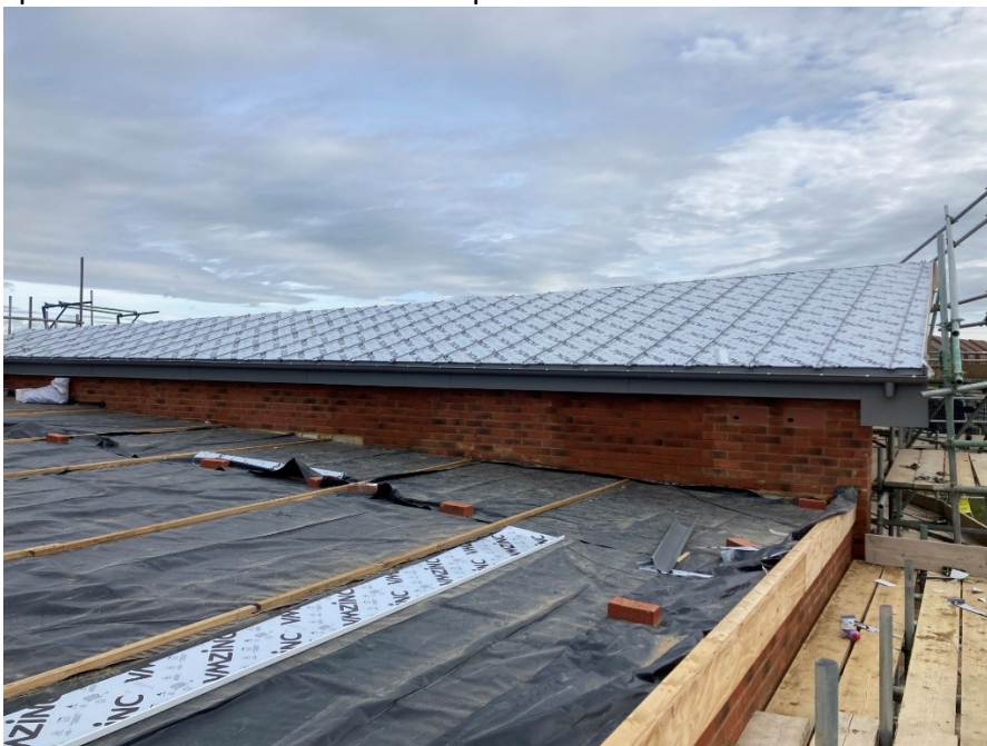
View taken from the top of the scaffolding looking over the roof showing completed zinc area and space where sedum roof will be planted
