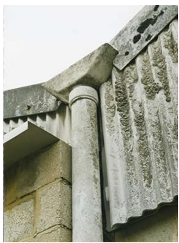
Asbestos cement downpipe, hopper and profile sheet
