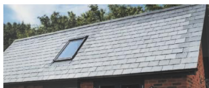
integrated solar and matching natural slates
