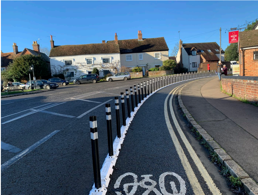
Figure 3-1: Pop up cycle lane on Tacks Lane (January 2022)
