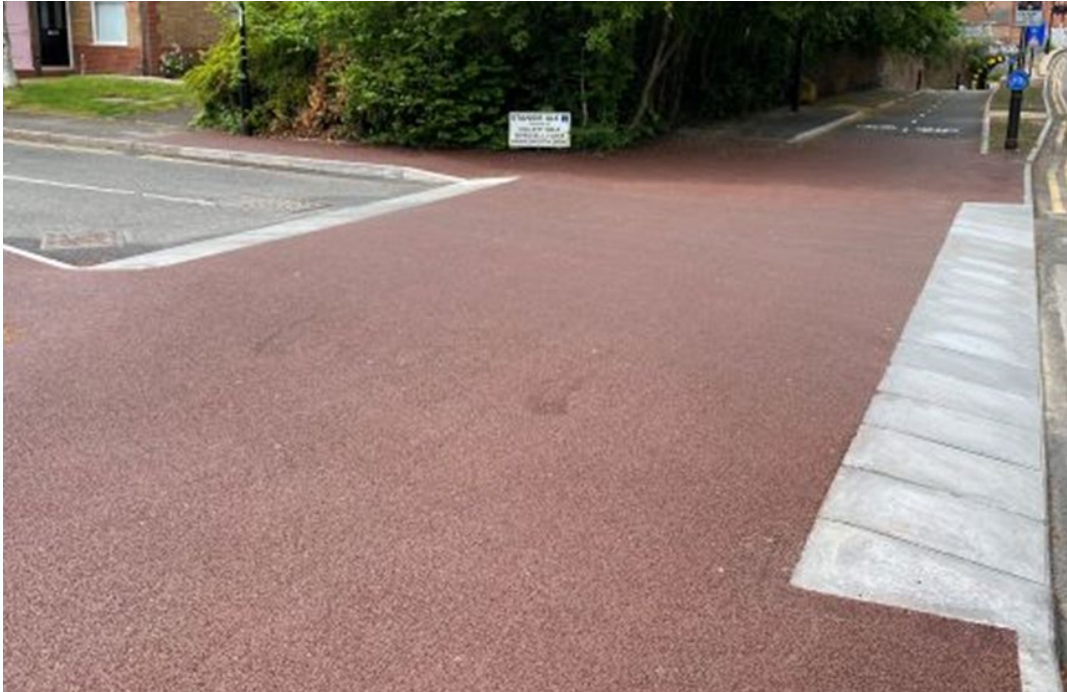
Figure 4-2: Continuous Footway Design (Credit Charcon UK)
