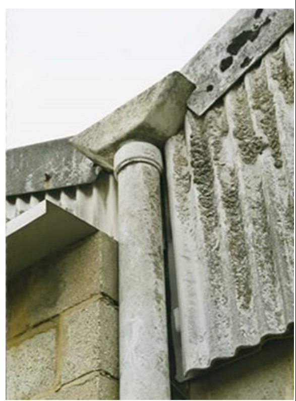
Asbestos cement downpipe, hopper and profile sheet
