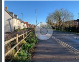
Poorly defined gateways
