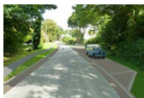
Defining parking bays
