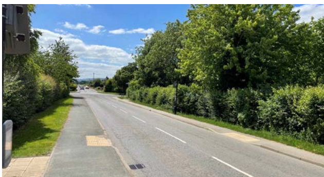
Photo 21. View south towards junction with Woodways
