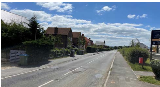
Photo 20. View south along Stanbridge Road
