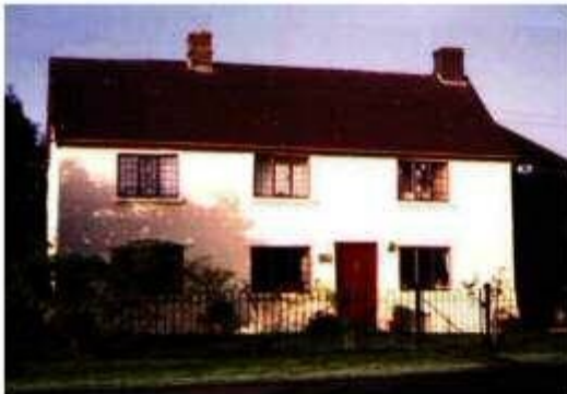
An early 19th century witchert house in Grendon Underwood, recently lime-rendered and lime washed after its pebble-dash had been removed.
