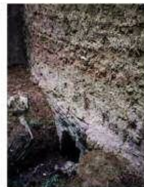
Newly rebuilt witchert wall over stream before trimming.
