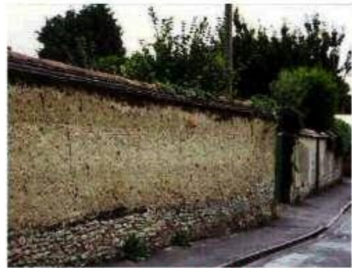
Witchert wall showing three berries above the grumplings. The coping is formed from plain and half round tiles.
