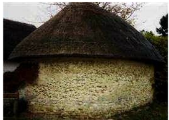
Small thatched witchert stable, the walls are pockmarked by masonry bees, but remain sound and dry under the overhanging thatch and above the unaltered stone plinth
