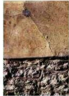
Cement mortar pointed grumplings and cement render. Cracks in both are drawing in water through capillary action. The moisture is unable to escape through dense render and cement mortar.
